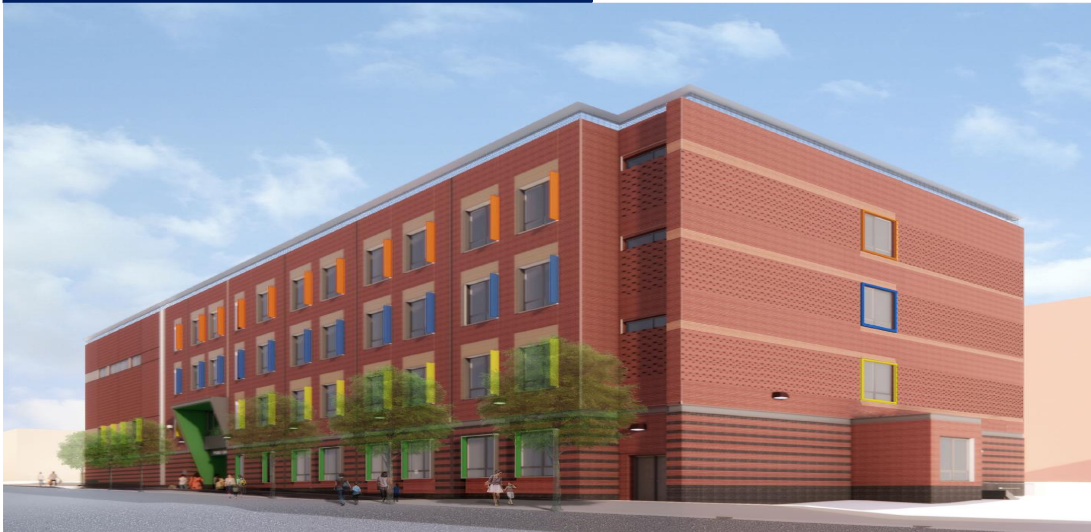
Q489 (PS 85 ANNEX) – 23-35 29 STREET – ANTICIPATED OPENING DATE: SEPTEMBER 2024 – TOTAL SEATS: 451
